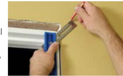
Lay Out Mitered Corners
