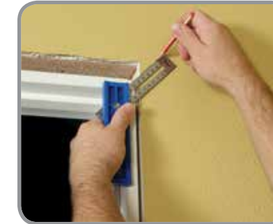
Lay Out Mitered Corners
