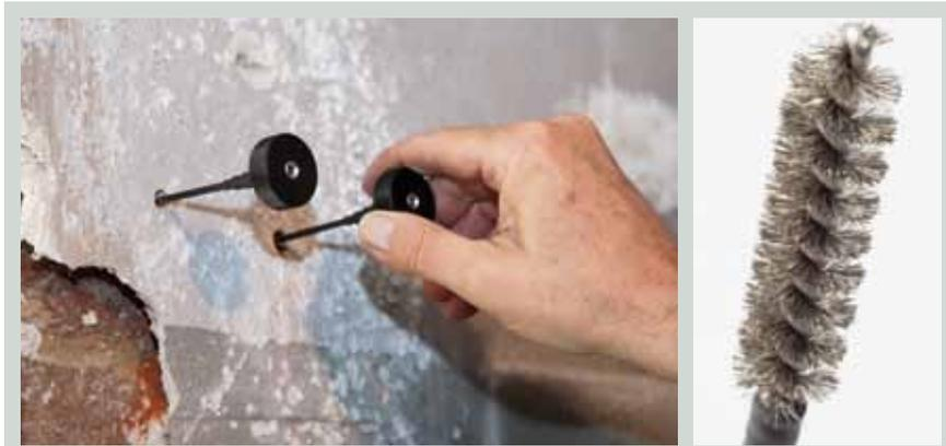
**APPLICATION** The brush electrodes are put into the pre-drilled hole
